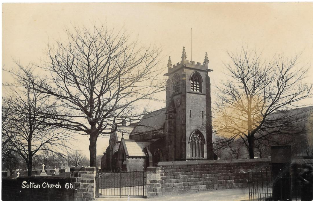
St. Thomas’s Church, Sutton (Photograph courtesy of Barry Durham)
