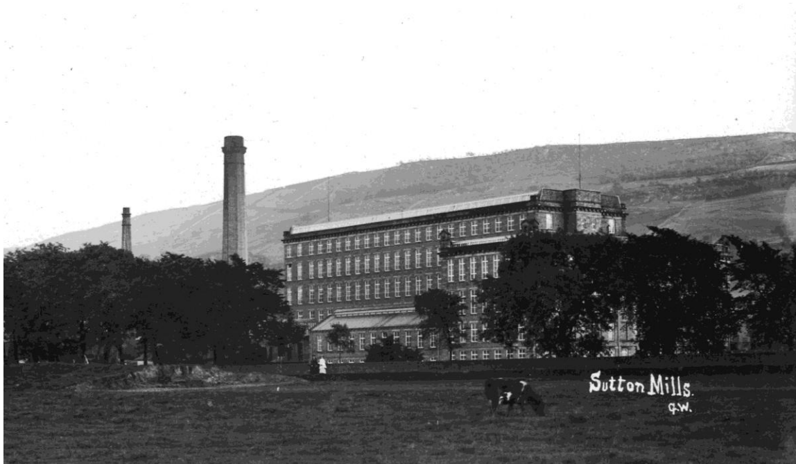
A George Whiteoak photograph of Bairstow's Mill, Sutton. Probably taken immediately prior to WW1. (By kind permission of Keighley and District Digital Archive)
